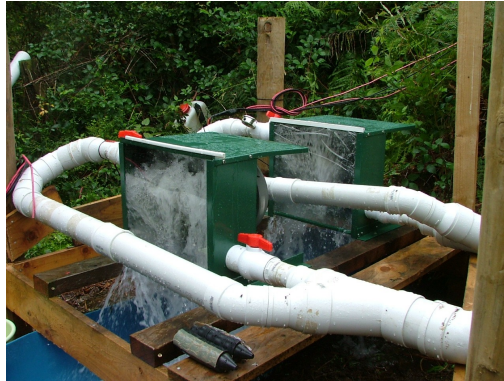
Low head install – 2 or more turbines
