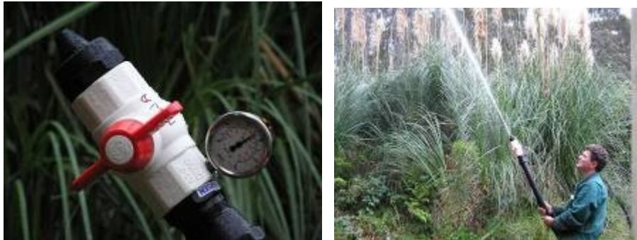
Cut jet and test flow rate with jet removed from turbine
