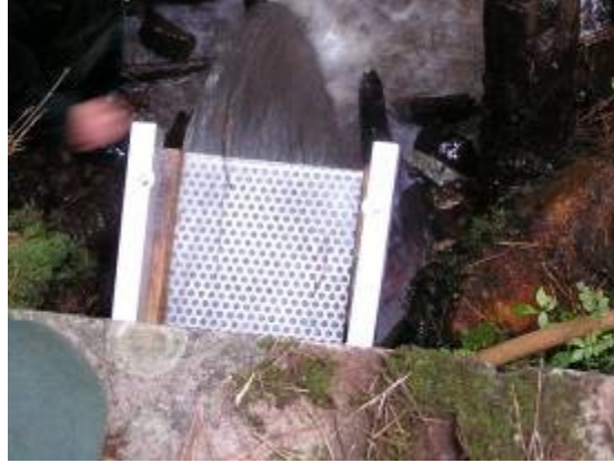
Perforated galvanized cable tray intake
